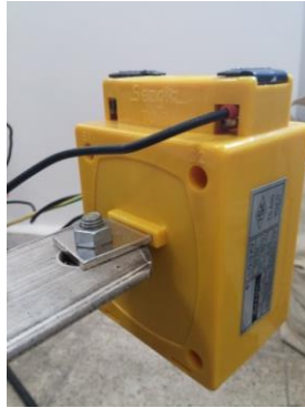
Figure 10. 10/5A current transformer
